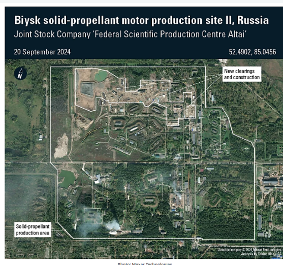
FIGURE 2 | Biysk II - solid-propellant facilities
